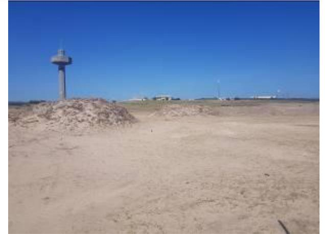
Image 12: Stockpiling of topsoil.
