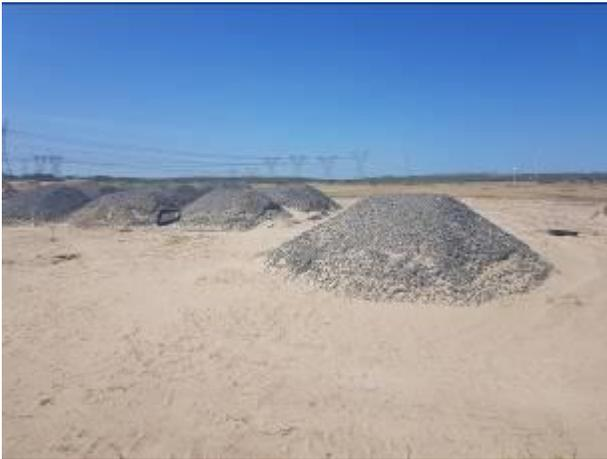
Image 13: Stockpiling of aggregate.
